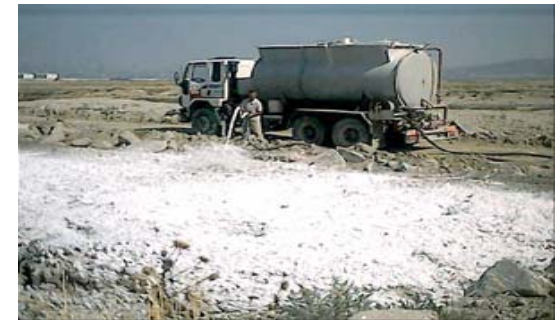
Covering over of a solid waste site with Alkeo-Hydrate disinfectant in solution form
